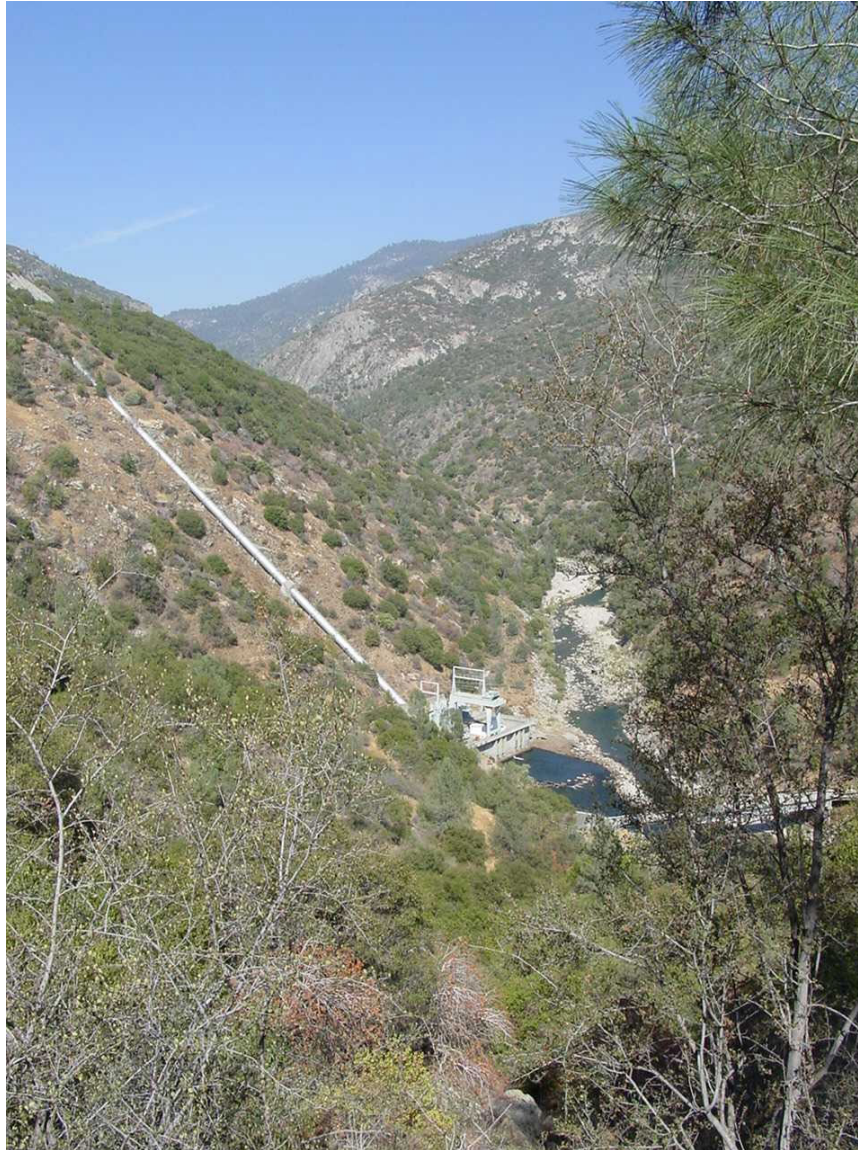
Photo 4. Mammoth Pool Powerhouse and Penstock (viewed from USFS Road 8S03).
