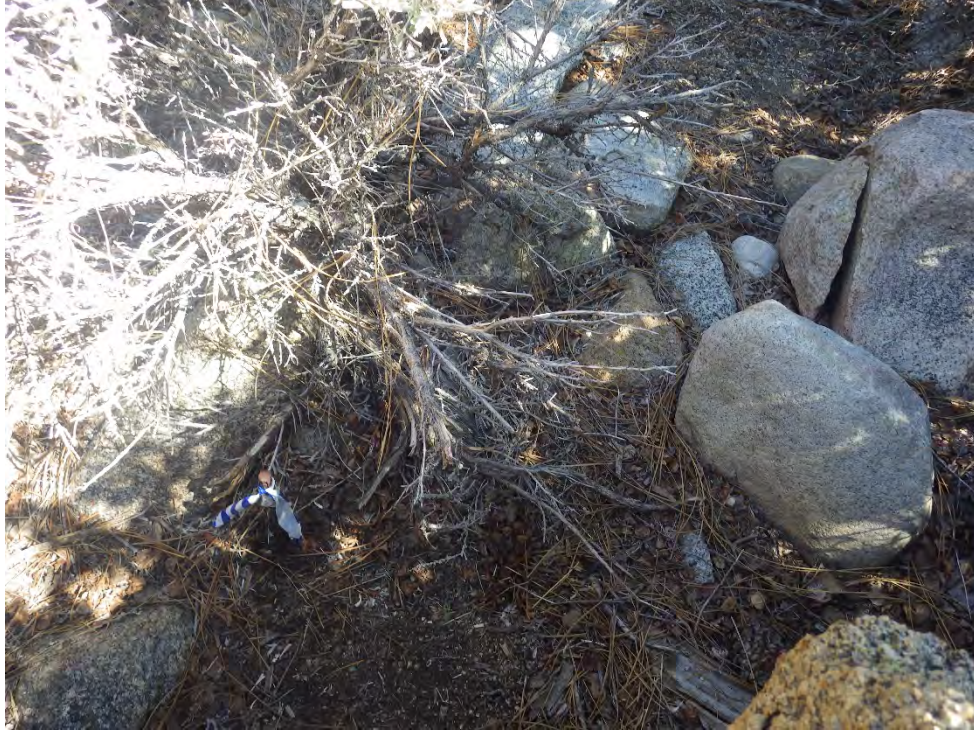
Figure A-27. Cross section 4.5 in August 2020, close up view of left bank pin.
