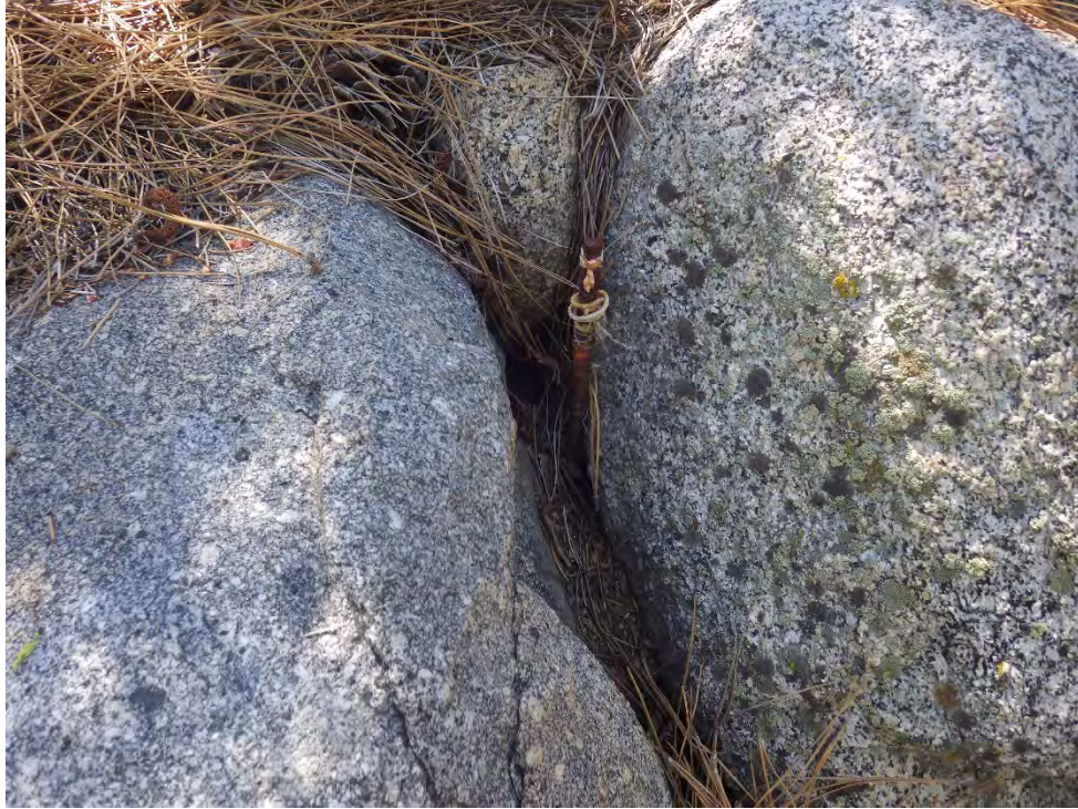
Figure A-17. Cross section 4.7 in August 2020, close up view of right bank pin.
